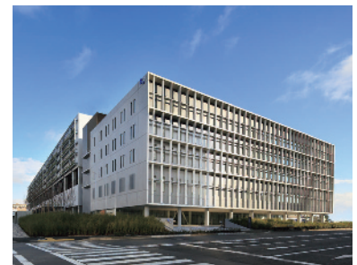
The Sagawa Tokyo Logistics Center (Koto-ku, Tokyo)
