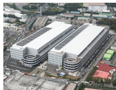
SG Realty Kashiwa equipped with solar power panels
